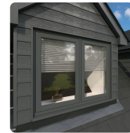
On timber cladding
