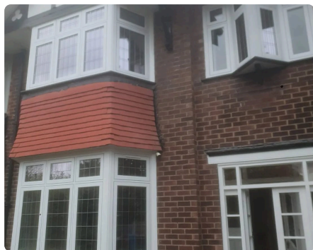
Leaded bay windows with Tudor detailing, 1930s semi
