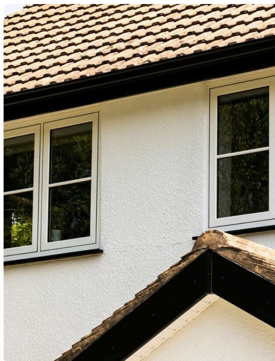
Cream flush sash windows on a period home
