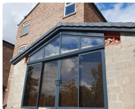
Corner bi-fold doors on a new-build extension
